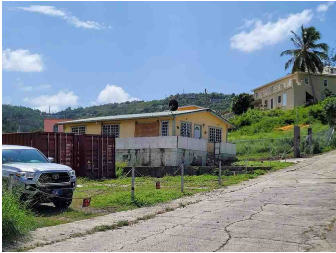
Parking Lot between structures
